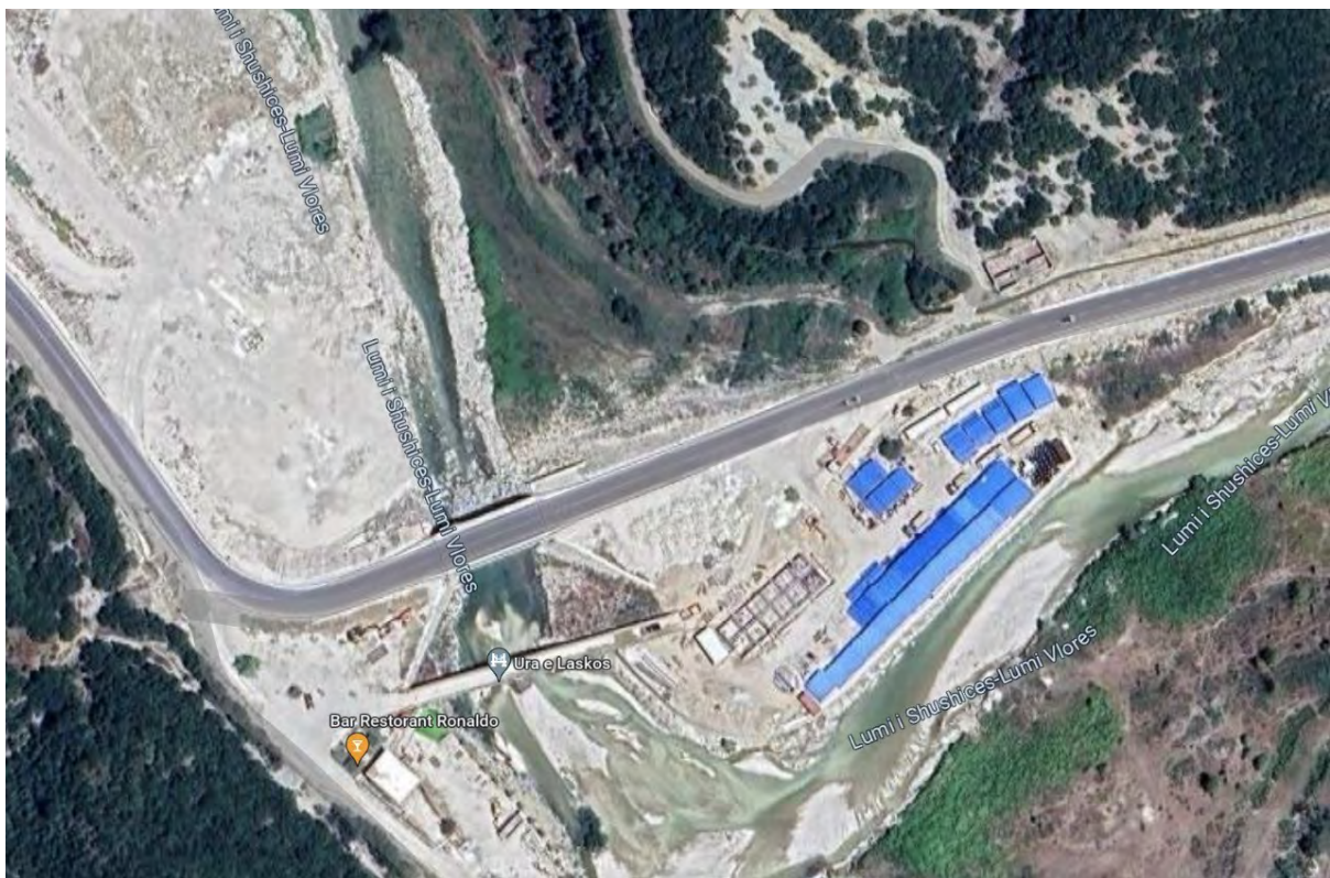
Figure 2: Storage Location at Lasko Bridge at the Shushica, partly build inside the national park. © Google Earth 2023
