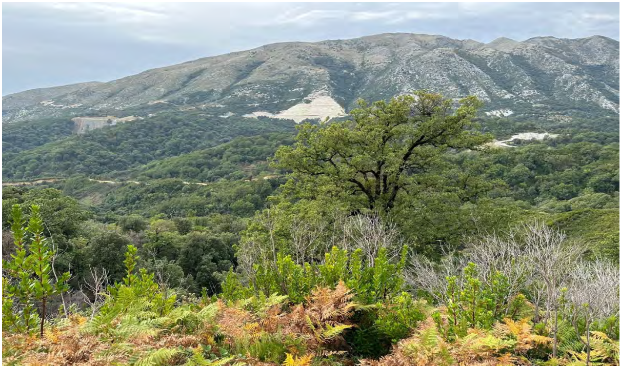
Figure 4: The construction of the pipeline route in the middle of the oak forest © Riverwatch
