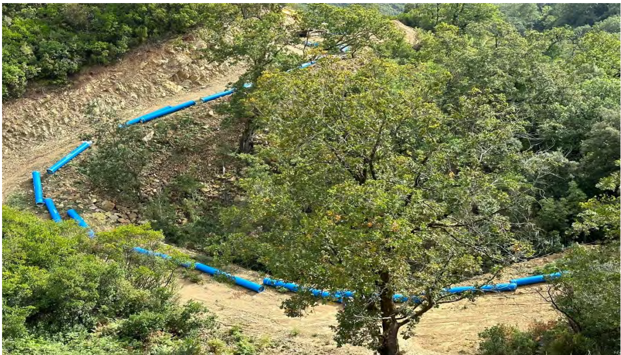
Figure 5: The pipes are already close to Kuc. Construction is ongoing © Riverwatch
